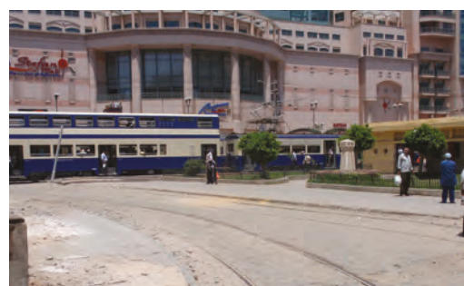
The original technological system of the substation (up) - in the photo, there is a substation similar to the one which must be upgraded after fire to recover one of the tram lines in Alexandria.
