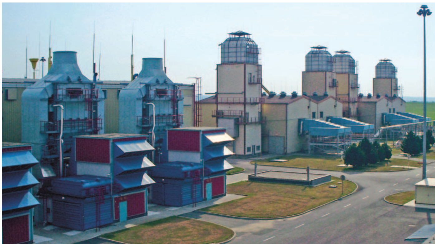
Kompressorová stanice 04, Ivanka u Nitry.
